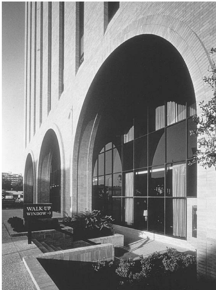
Figure 11-20 United Bank Tower in Austin, Texas—Zapalac and Associates Architects. (Photo courtesy BIA.)
